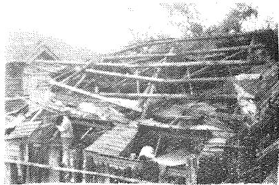
高雄員工宿舍被毀情形 Destroyed dormitory of railway-workers at Kaohsiung.
