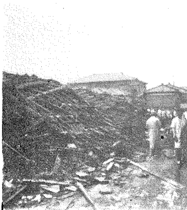
碼頭工人宿舍倒塌 Destroyed dormitory of the wharf workers.
